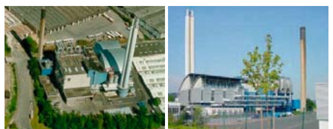
12 Hagen refuse incineration plant • MVA Hagen
